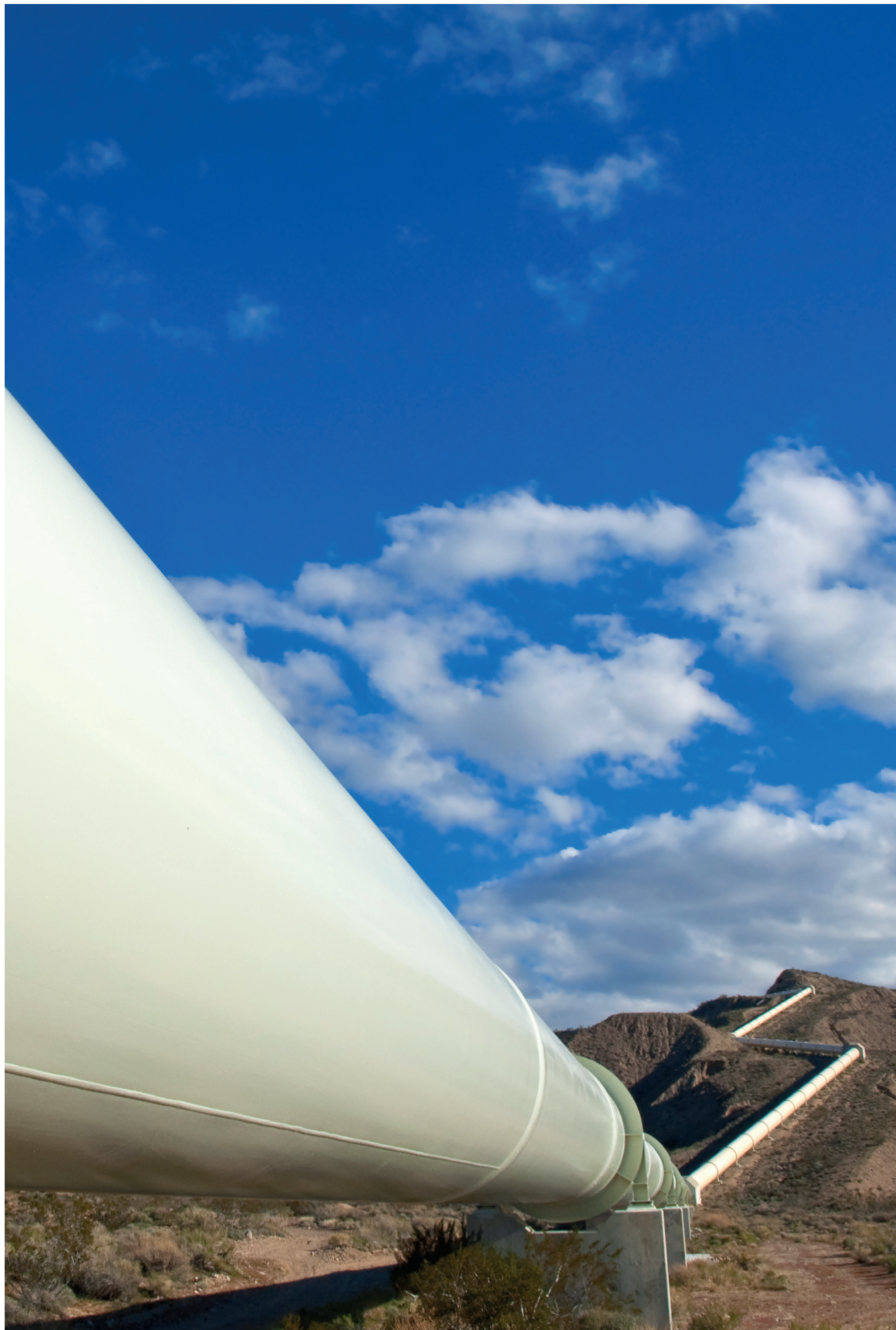
— North Stream Pipeline —
